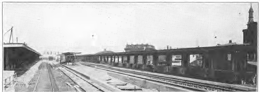
Passenger Station, Covington, Ky., showing three covered platforms
